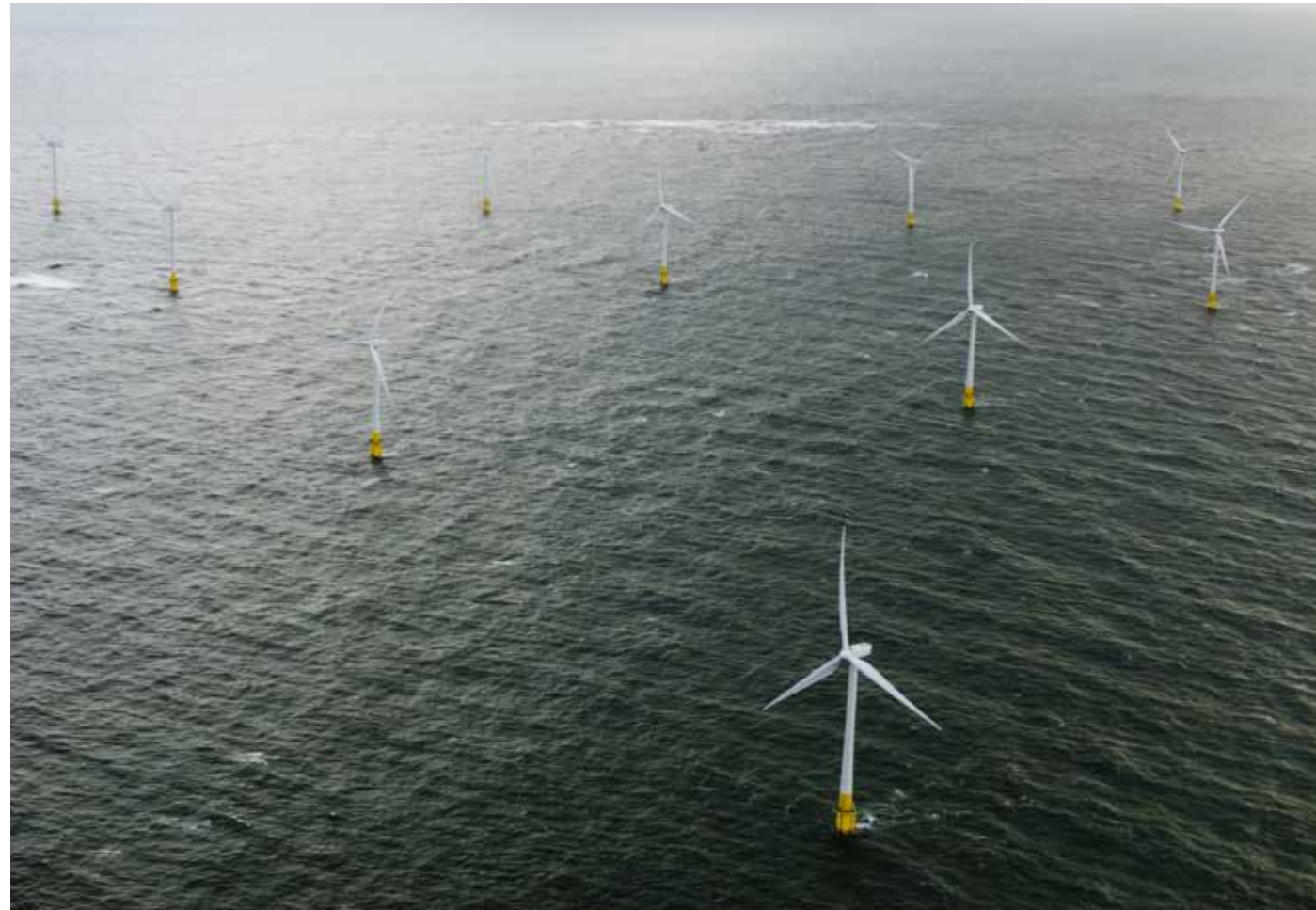
Aerial view of offshore windfarm, wind turbines at sea, UK. © David Tipling/FLPA
