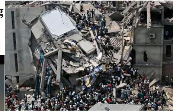
Rescue workers trapped under rubble at the Rana Plaza building after it collapsed, in Savar, Dhaka on April 24 last year. Photograph: © Andrew Biraj/Reuters
