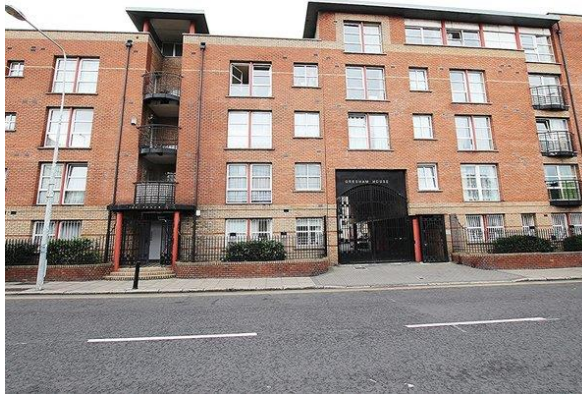
Marginally Engineered Structure
