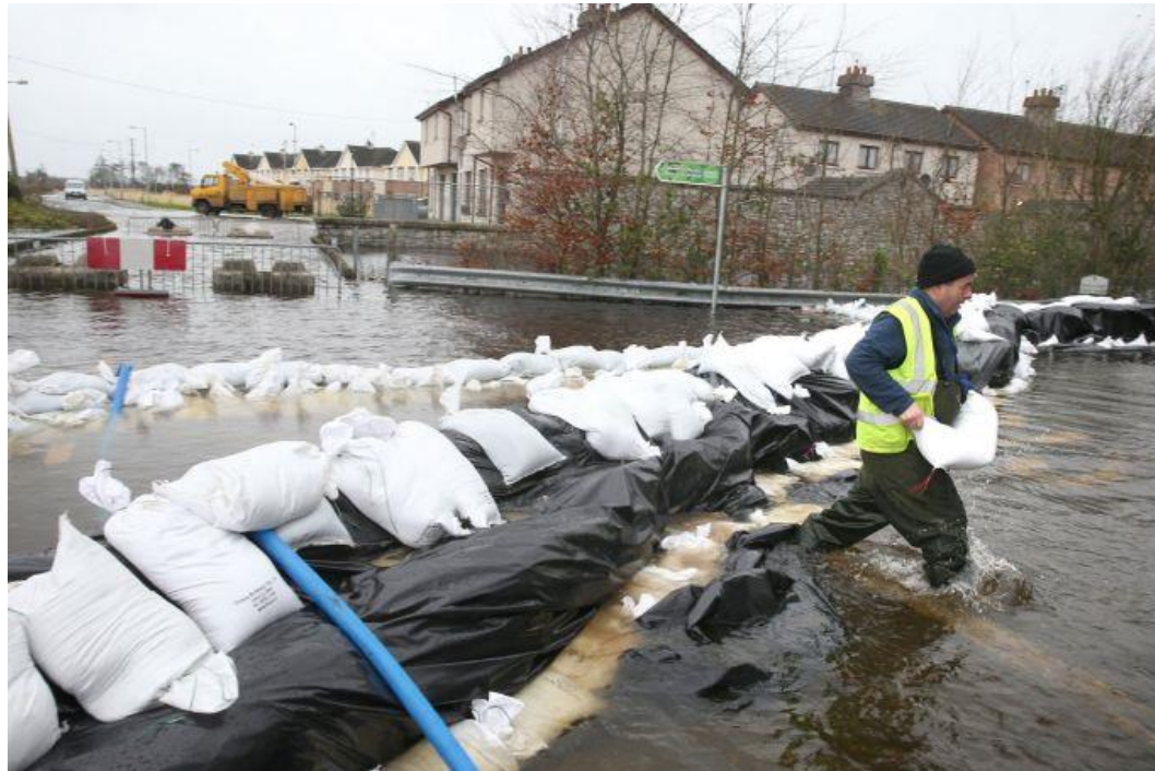
Local Councillor Kevin Moran helps with flood defences in Athlone. Photograph: Brian Lawless/PA Wire
